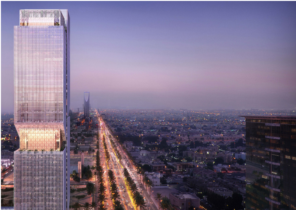
Alinma Bank New Headquarters
