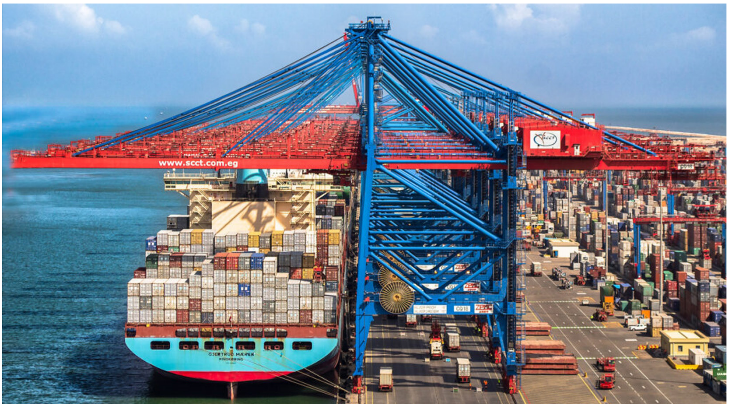
Portsaid East Container Terminal
