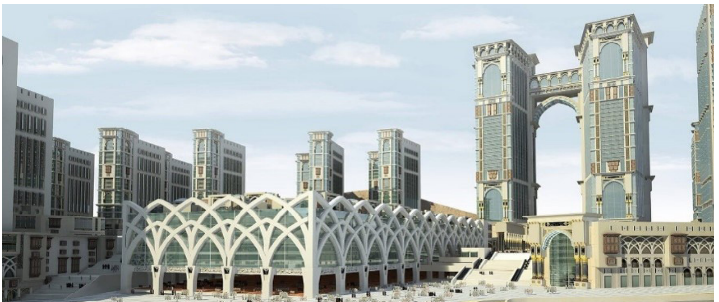
Jabal Omar Development Project (Phase IV)
