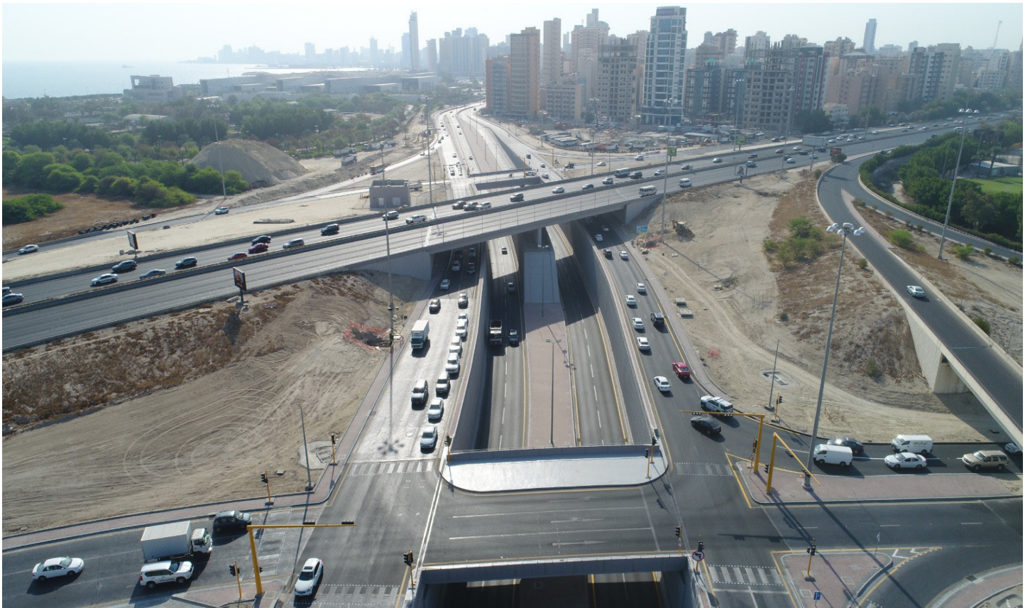
Design of Three Troughs and Three Pump Stations for Cairo Street, RA/200
