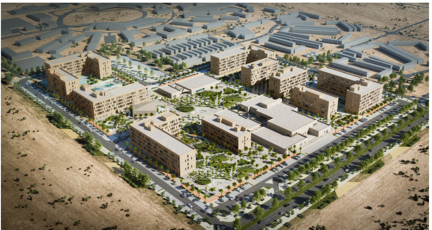
1600 Staff Accommodation Units (SAU) for ENEC
