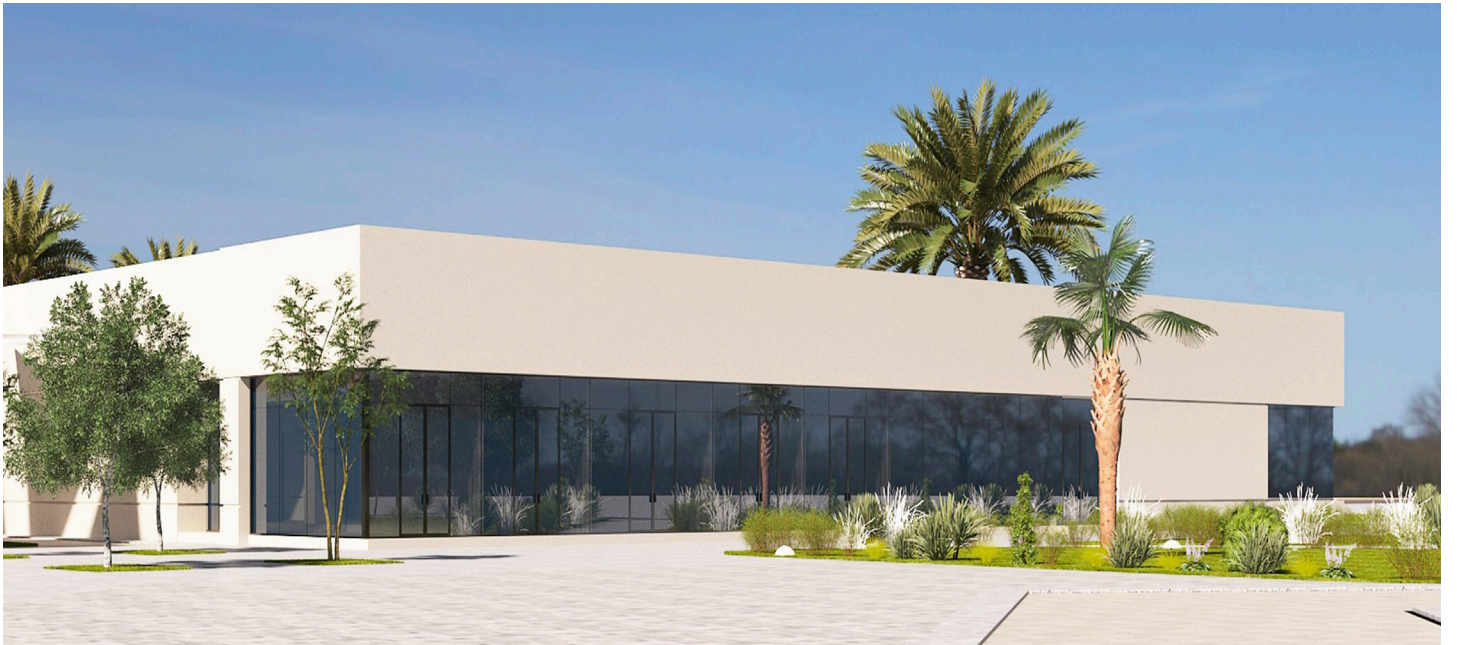
1600 Staff Accommodation Units for ENEC
