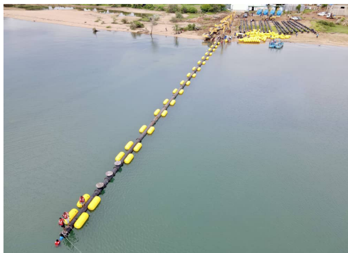
Karonga Town Water Supply Project
