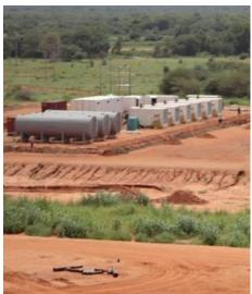
(supplied and installed by others), instrumentation and telecommunication system inclusive of fiber optic cables connecting wellheads to the main plant control room, related civil works. FSF works also included 5 flow lines of 6" diameter, insulated and underground of total length of around 8 km.
